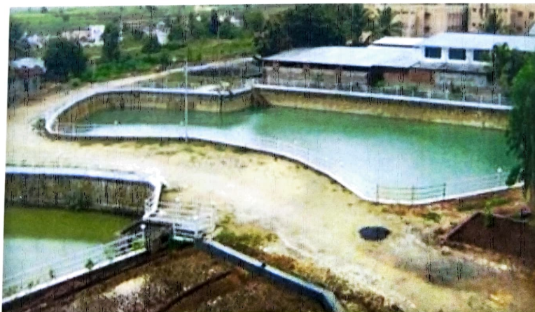
Fig:4.4 Rain water harvesting arial view
